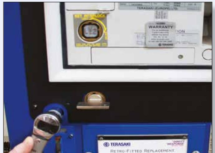
Withdrawable functionality and safety interlocks of original devices can be retained and improved. Fixed pattern devices can even be replaced with withdrawable devices.
