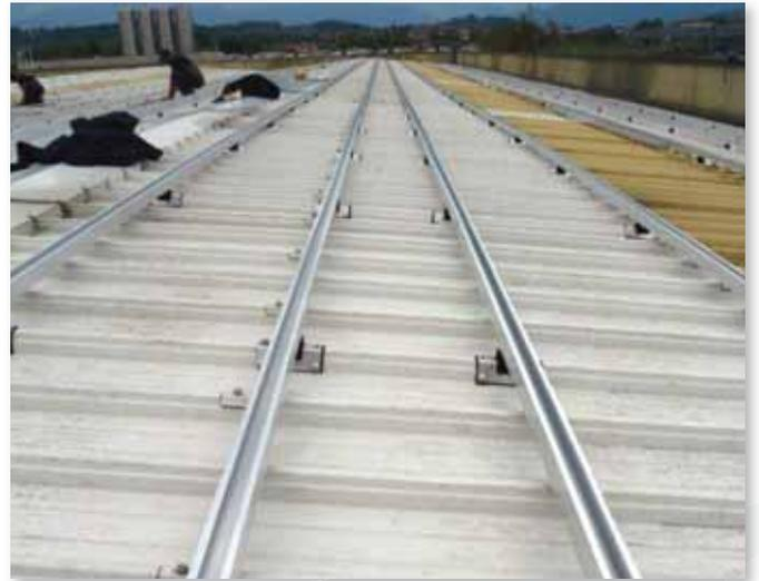
Metal decking roof. Application with brackets as per drawing FVT95XX.
