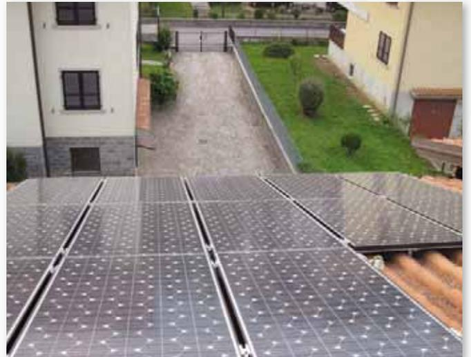
Sloping roof with tiles. Application with stainless steel adjustable bracket FVT1256.
