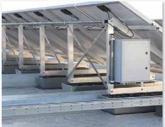
Triangle single vertical at 30° with ballast tanks.
