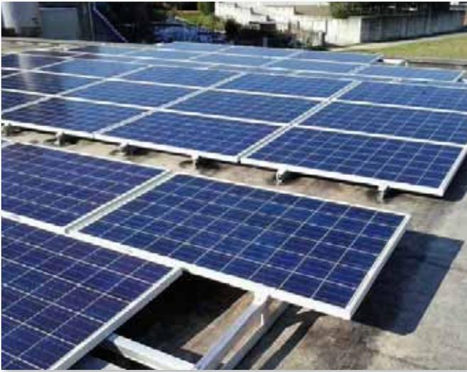
Triangle triple horizontal ballasted.
