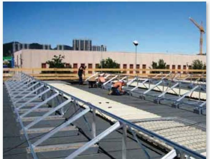
Flat industrial roof with sheath. Application with ballast tanks FVT1455 and triangles at 30° FVT1511.
