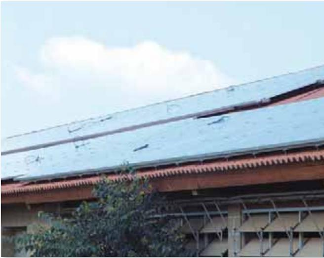
Sloping roof- asbestos recovery. Application with mill screws for wood FVT1315.
