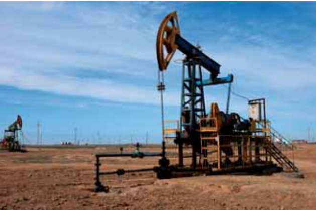
>300 VLT® Advanced Harmonic Filters installed at decentral oil pumping stations. Ensures 24hour/day pumping.
