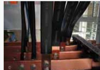
**$\Omega$  FLEX** bars are made of red copper laminates (Cu ETP) coated with an extruded PVC insulation which gives excellent electrical insulation even in the presence of dampness, aggressive temperatures and environments.
