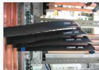
$\Omega$  LINK is a ready-to-use flexible prefabricated shunt made in tinned copper braid, coated with PVC insulation.
