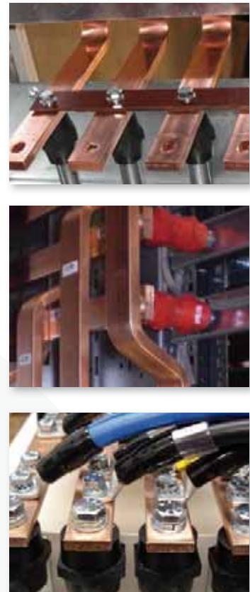
The "stand off" insulator is used as an insulating support for active conductors to guarantee excellent electrical insulation capability; it can be used as a support for electrical devices, giving high mechanical resistance values, as well as a spacing and/or stiffening element of a system made of conductor bars (copper and/or aluminium).
