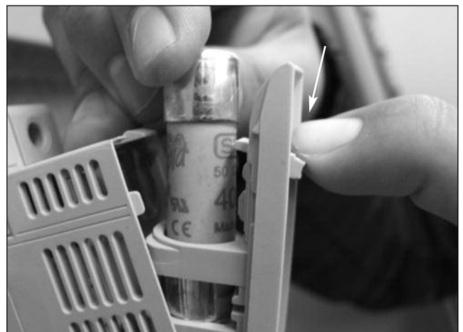
4. Pressing downwards the fuse-holding clip to insert or remove the fuse
